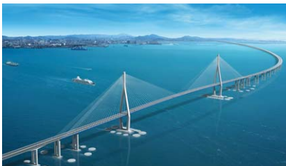
Incheon Bridge, opened in October 2009 World's 5 th longest cable-stayed bridge
